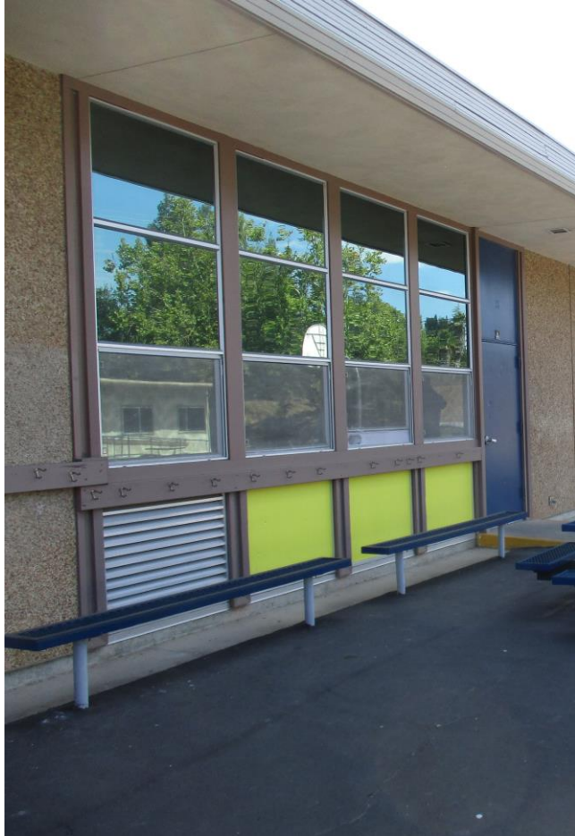
Typical Existing Façade
