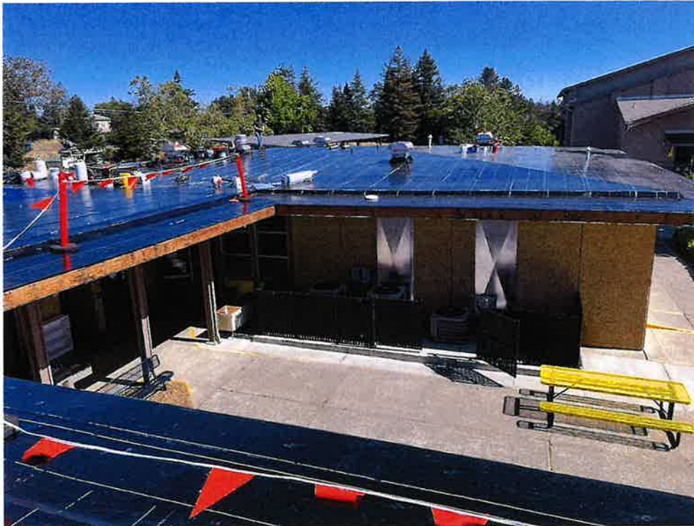
Another View of Building A Roof with modified base sheet.
