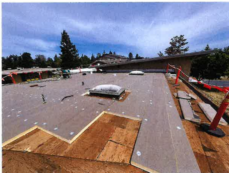
Installation of 3.5 inch foam insulation to roof decking
