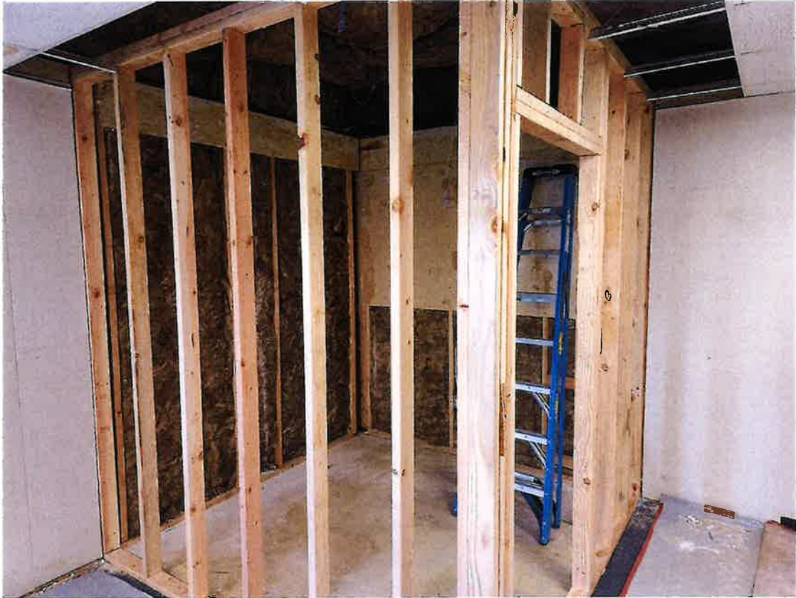
Restroom Framing at Rm 24 Gravenstein
