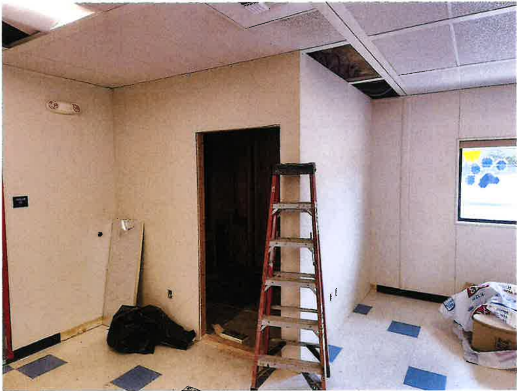
Restroom with Tackwall at Rm 22 Gravenstein
