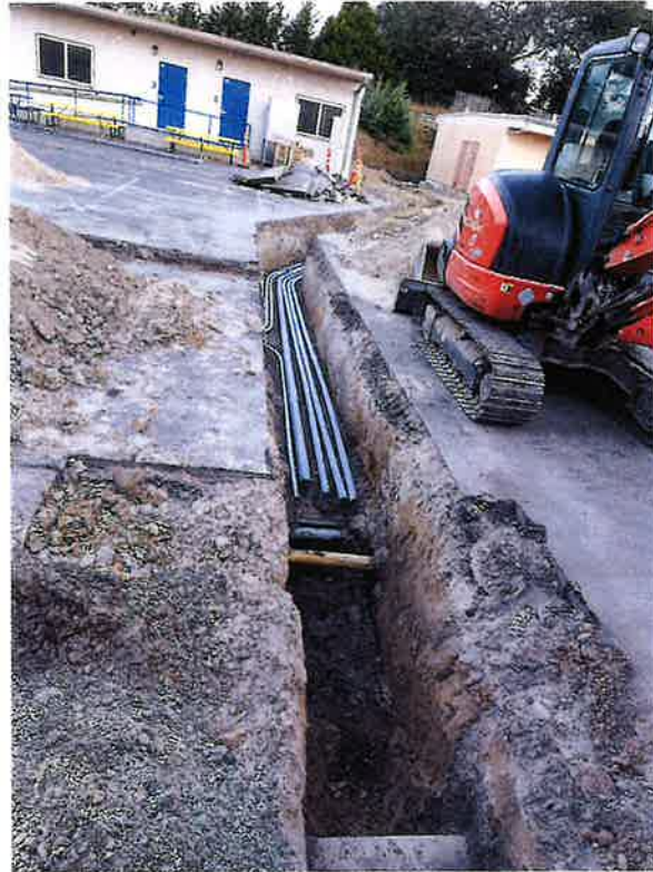
Electrical Utility trenching for modular
