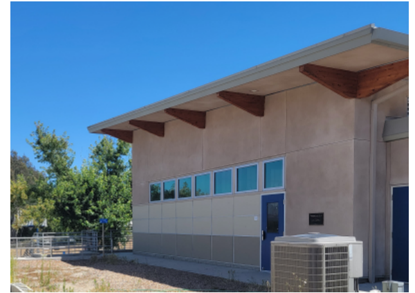
Exterior of Building
