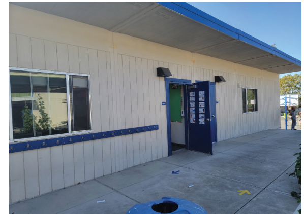
Exterior of Building
