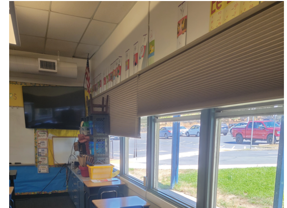
Classroom windows/window coverings
