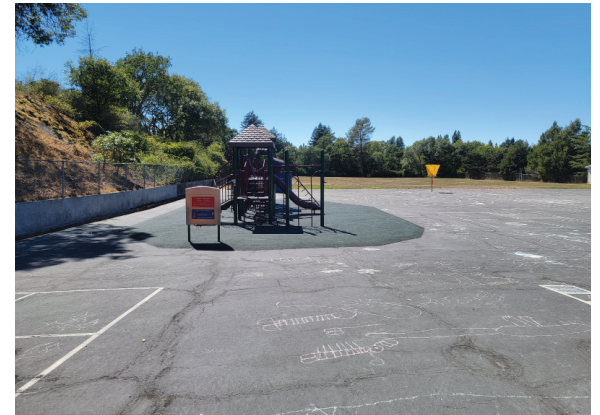
AC paving at playground
