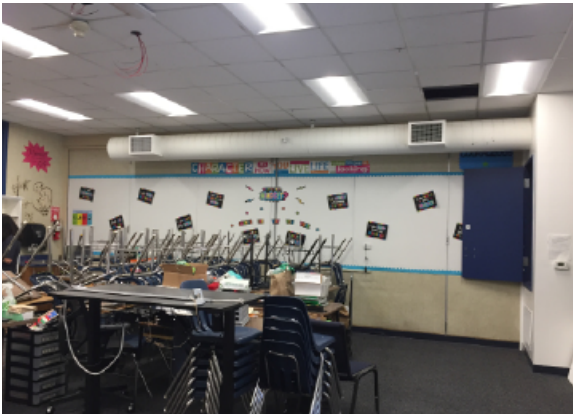
Classroom Interior - Operable Wall & Mechanical
