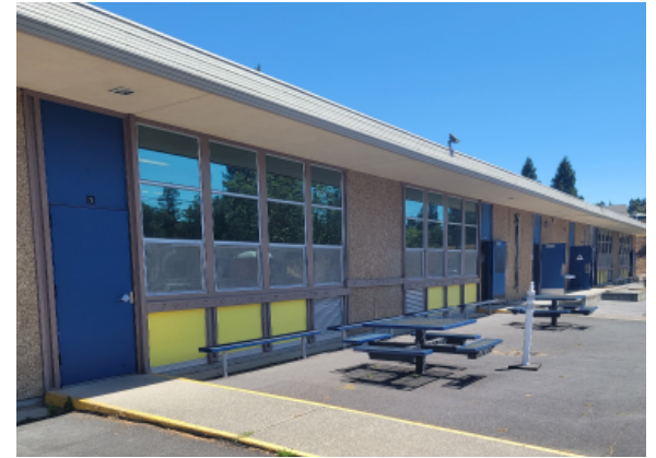
Exterior of Building
