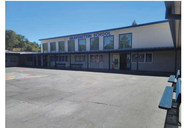
Exterior of Building
