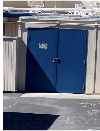
Utility Transformer Room
