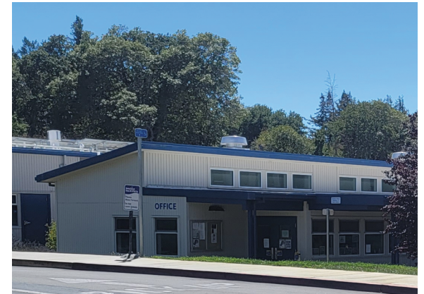
Exterior of Building
