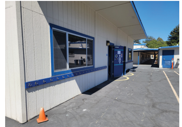
Exterior of Building
