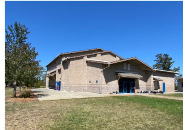
Exterior of Building
