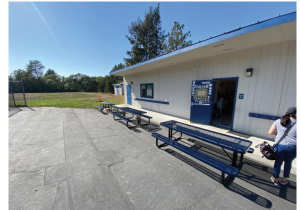
Exterior of Building
