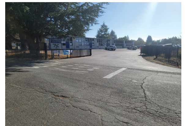
Arrival to site - missing safe pedestrian path
