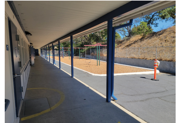
Exterior of Building
