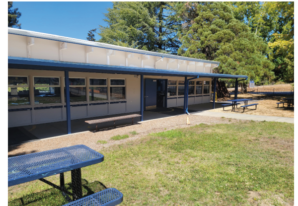
Exterior of Building
