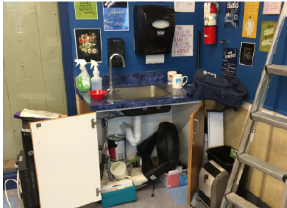
Classroom Sink - Not Accessible
