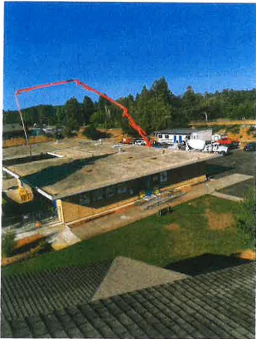
Concrete Pour with Concrete Pump for Condenser Pads.
