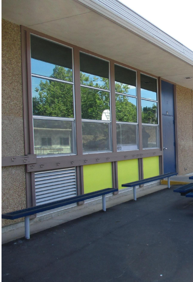
Typical Existing Façade
