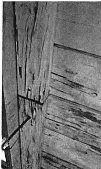
DRY ROT AT SIDING TRIM OBSERVED PRIMARILY AT BUILDINGS C, AND D
